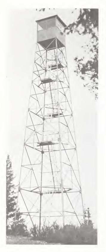
Figure 49. San Mateo lookout tower (Aermotor MC-40), constructed in 1934 on Cibola National Forest, New Mexico. Photograph made by W. E. Wiltbank in 1945 (U. S. Forest Service 435133).
